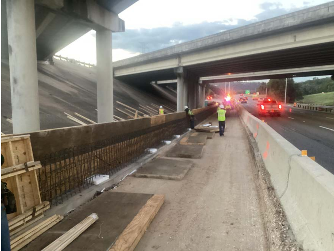
Loop 360 Underpass November 2023
