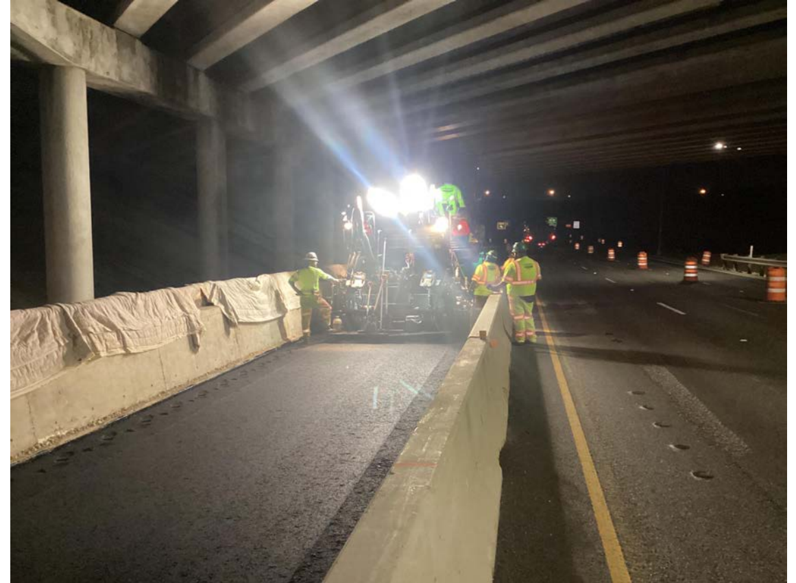
Inside Widening at Loop 360 November 2023
