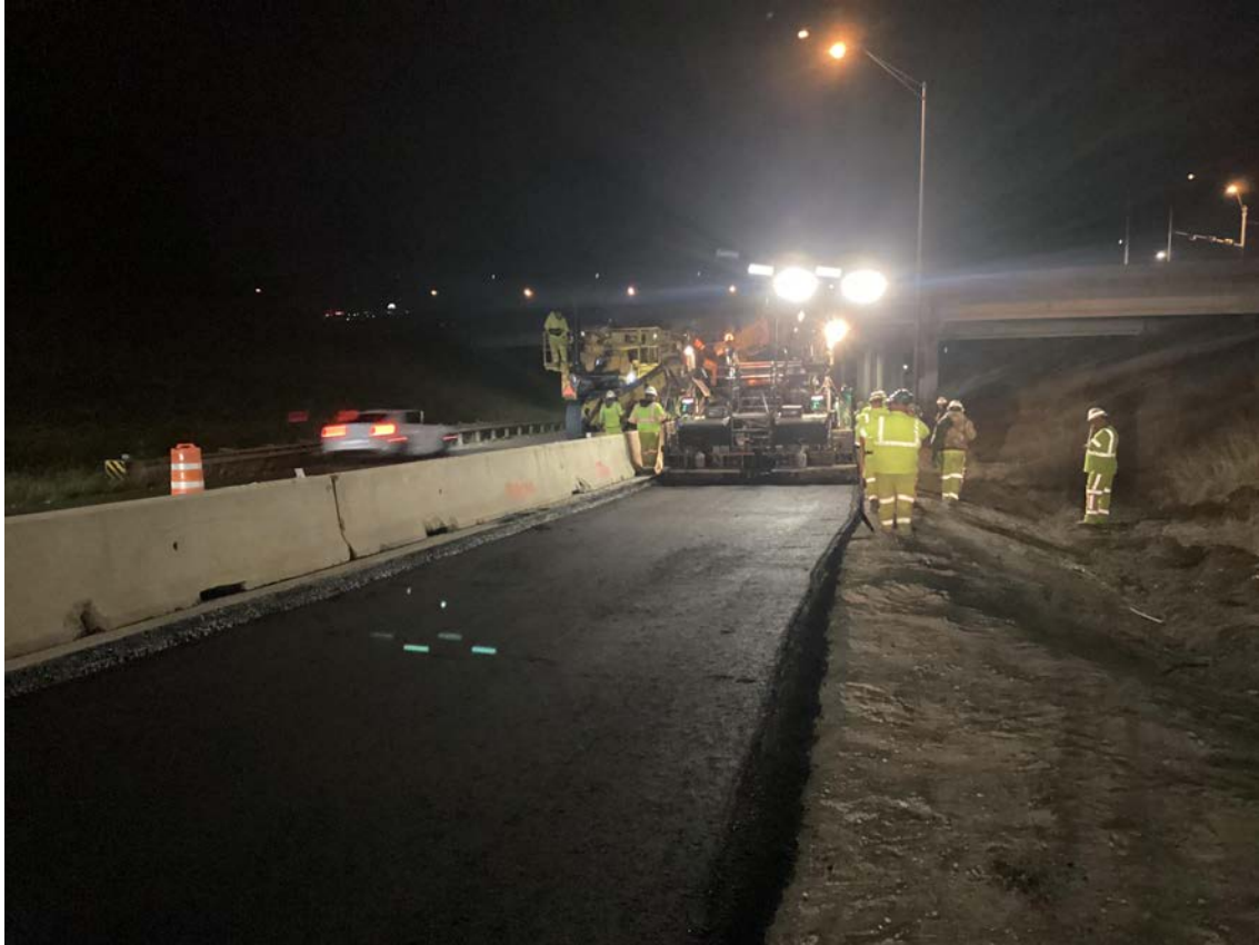
Outside Widening at Loop 360 October 2023
