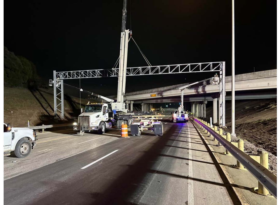
Loop 360 Underpass November 2023
