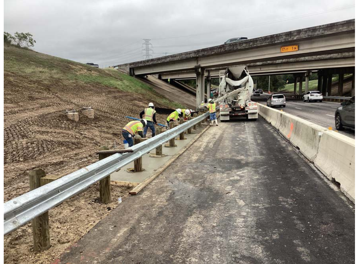
Loop 360 Underpass November 2023
